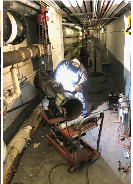
expansion joint with a torch and hanging rigging equipment to safely remove it.
